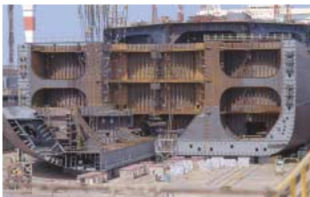
Double-hull structure
