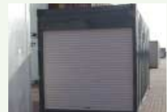
Setting up a garage made from a recycled container
