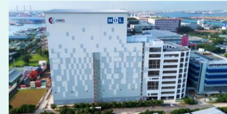
Energy-efficient refrigerated warehouse (Singapore)
