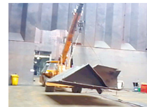
Dismantling operations in cargo hold
