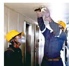
Removal of hazardous substances before dismantling
