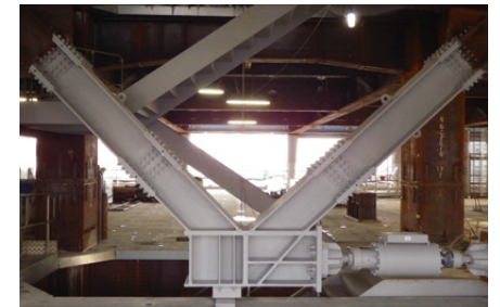
Vibration control structure in Shin Daibiru under construction
