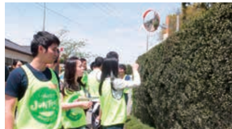
Examining traces of the flood damage on a hedge
