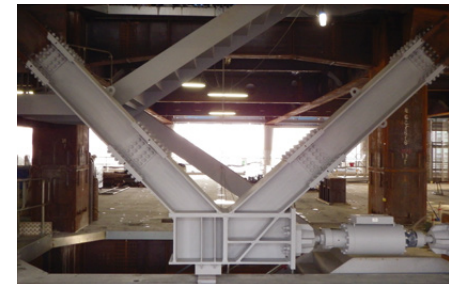
Vibration control structure in Shin Daibiru under construction
