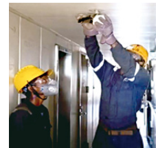
Removal of hazardous substances before dismantling
