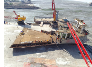
Dismantling operations after the vessel is pulled ashore
