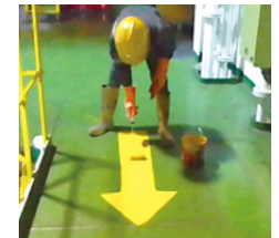
Renewal and repainting of escape routes
