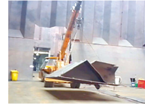
Dismantling operations in cargo hold
